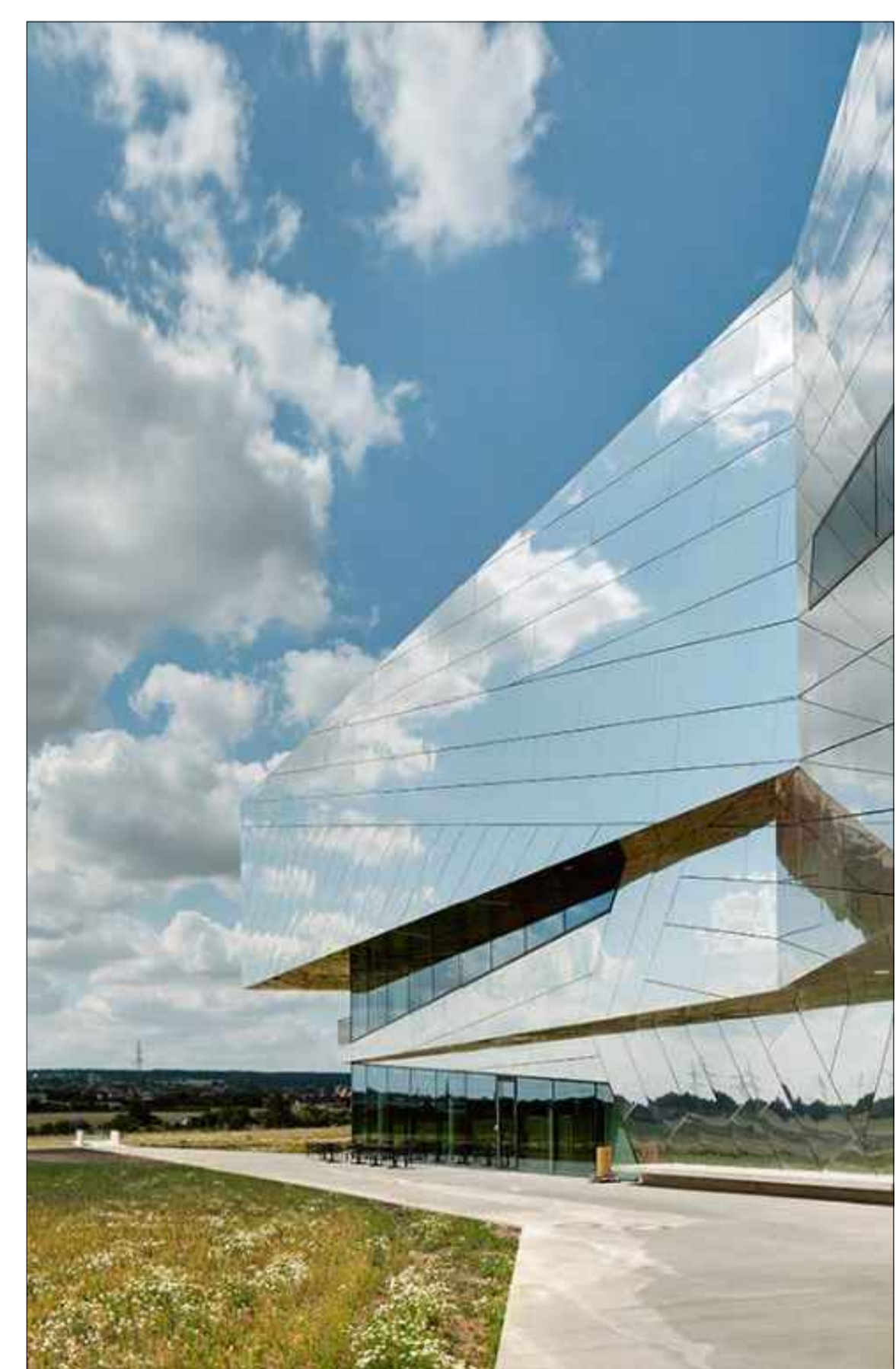
PHOTOGRAPHS SHOWING THE ALUCOBOND CLADDING PANELS AT THE SCHONINGER SPEARS BUILDING (GERMANY) (Paläon, Schöninger Speere)
