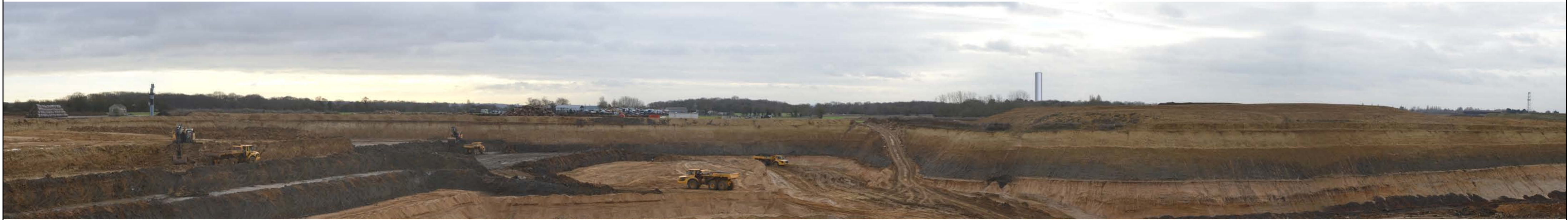
Viewpoint 4 - Taken from Cuthedge Lane, looking south-west towards the site. Stack at 108m AOD (58m above the surrounding ground level of 50m AOD). Note: Regardless of proposed landform and planting associated with restoration of quarry.
