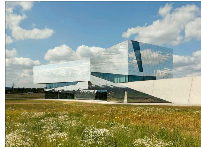
PHOTOGRAPHS SHOWING THE ALUCOBOND CLADDING PANELS AT THE SCHÖNINGER SPEARS BUILDING (GERMANY) (Paläon, Schöninger Speere)
