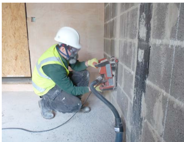
Figure 4 Wall chasing using on-tool extraction
