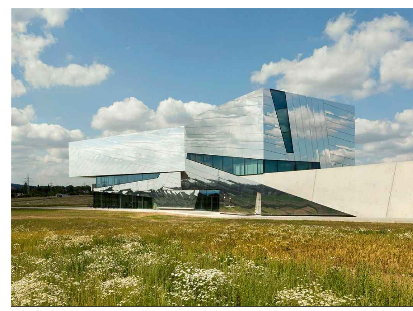
PHOTOGRAPHS SHOWING THE ALUCOBOND CLADDING PANELS AT THE SCHONINGER SPEARS BUILDING (GERMANY) (Paläon, Schöninger Speere)
